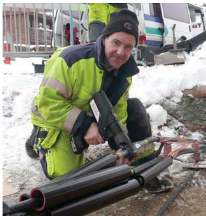
Crimping with Elpress crimp tool PVL1300.
