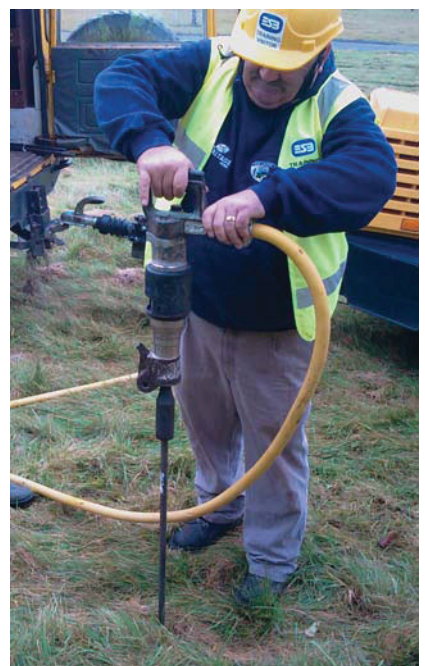
The driving down has started.
