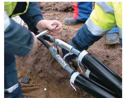
Bolts are tightened using a wrench. It is also possible to use a battery operated wrench.
