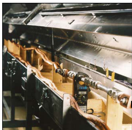
Testing of connections at the Elpress laboratory.
